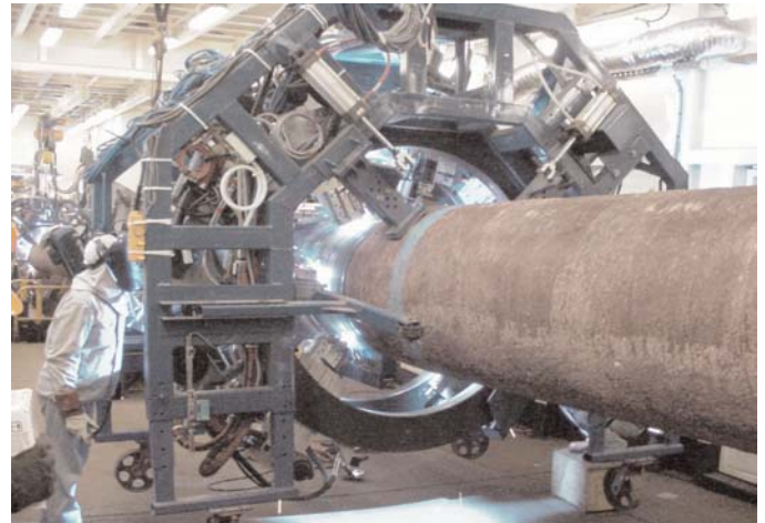
JAWS on Derrick / Lay Barge KP1
