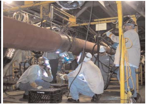
JBBS on Derrick / Lay Barge, DB16
